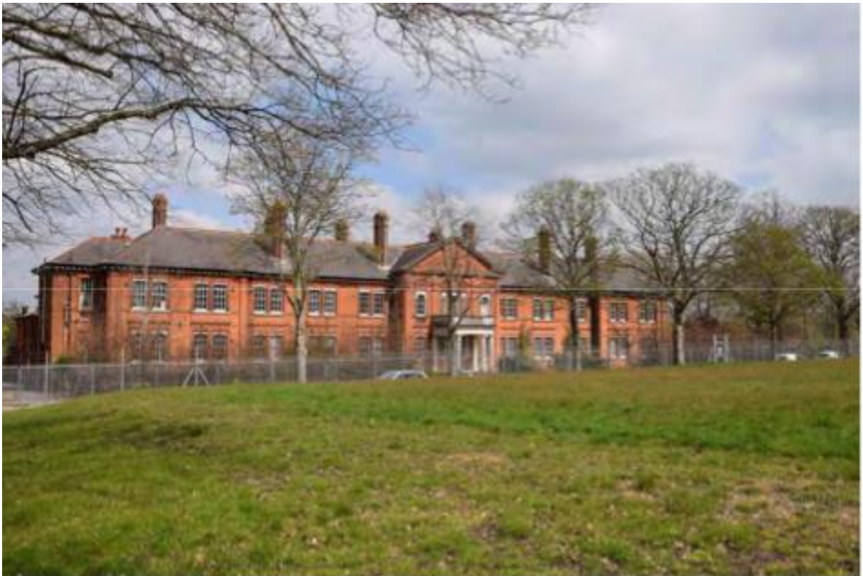
View from the south-west of the Headquarters Building
